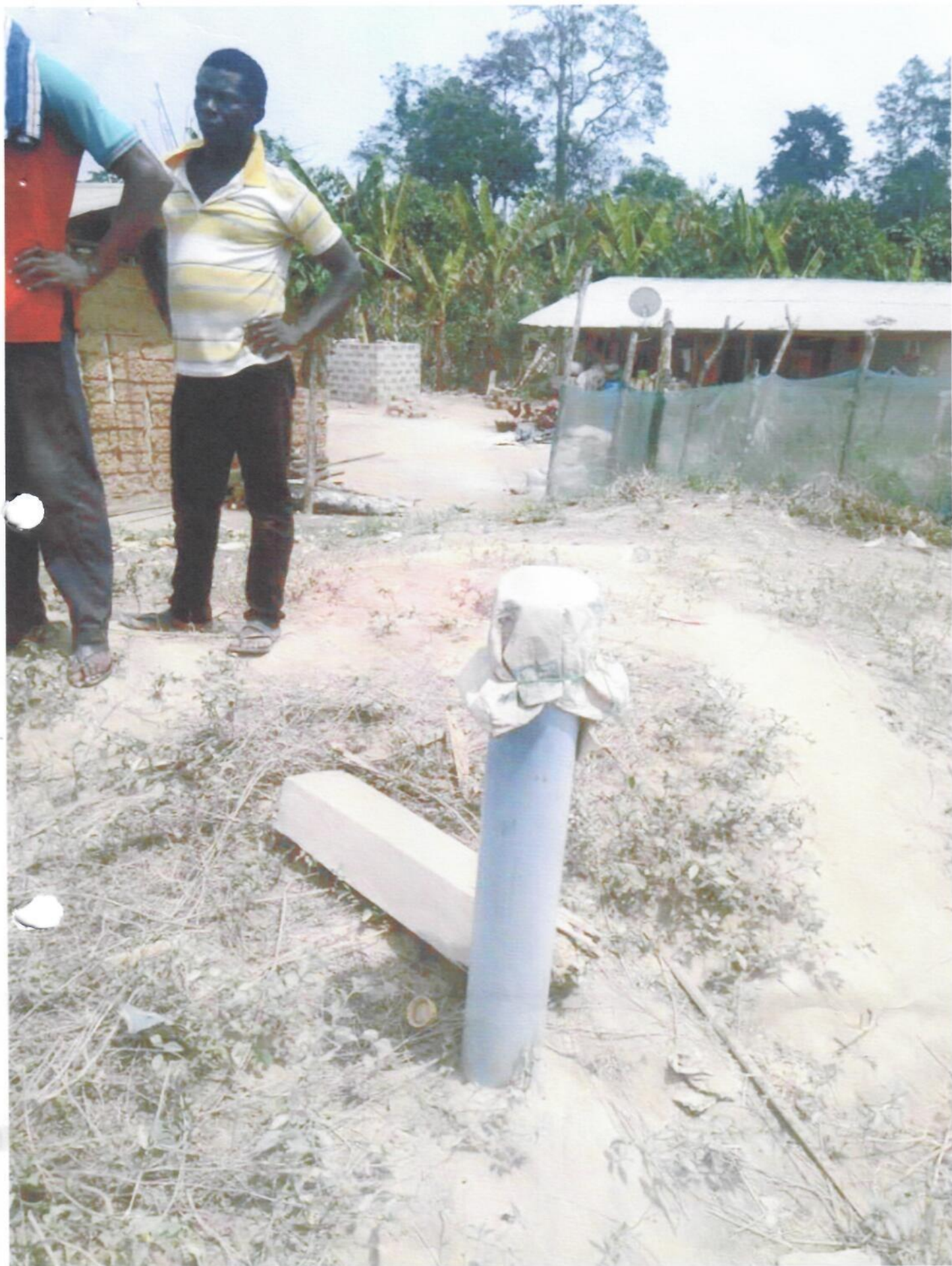
Appendix 'C1' — 'Borehole' without AfriDev Handpump ① purported to be in use © Yawobiri
